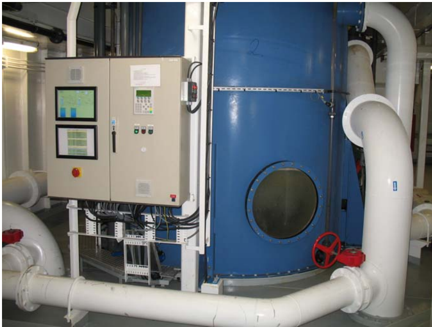
Figure 11. Water treatment unit onboard one well boat designed for closed transport. Photo: Kai Sørensen (NIVA).
