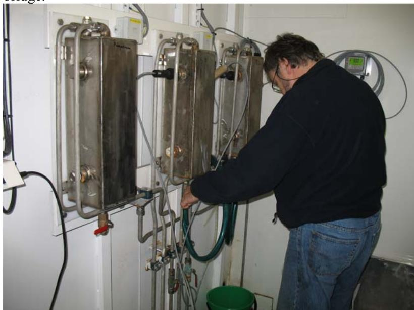
**Figure 10.** Water sampling from units leading water from two fish wells and outside water into a central monitoring and sampling unit onboard a well boat designed for closed transport. Photo: Trond Rosten
